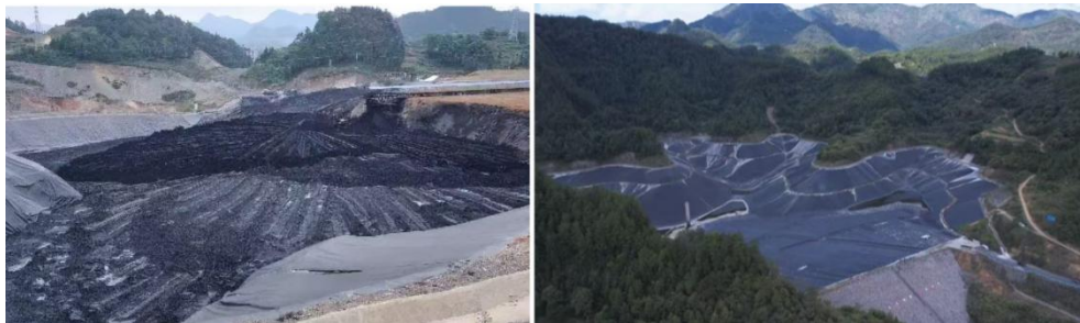
Figure 1.2: Open-air Storage of Manganese Slag
