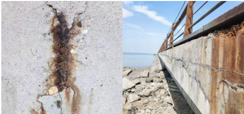
Figure 2.25: Morphology of Concrete Subjected to Long-term Chloride and Sulphate Attack
