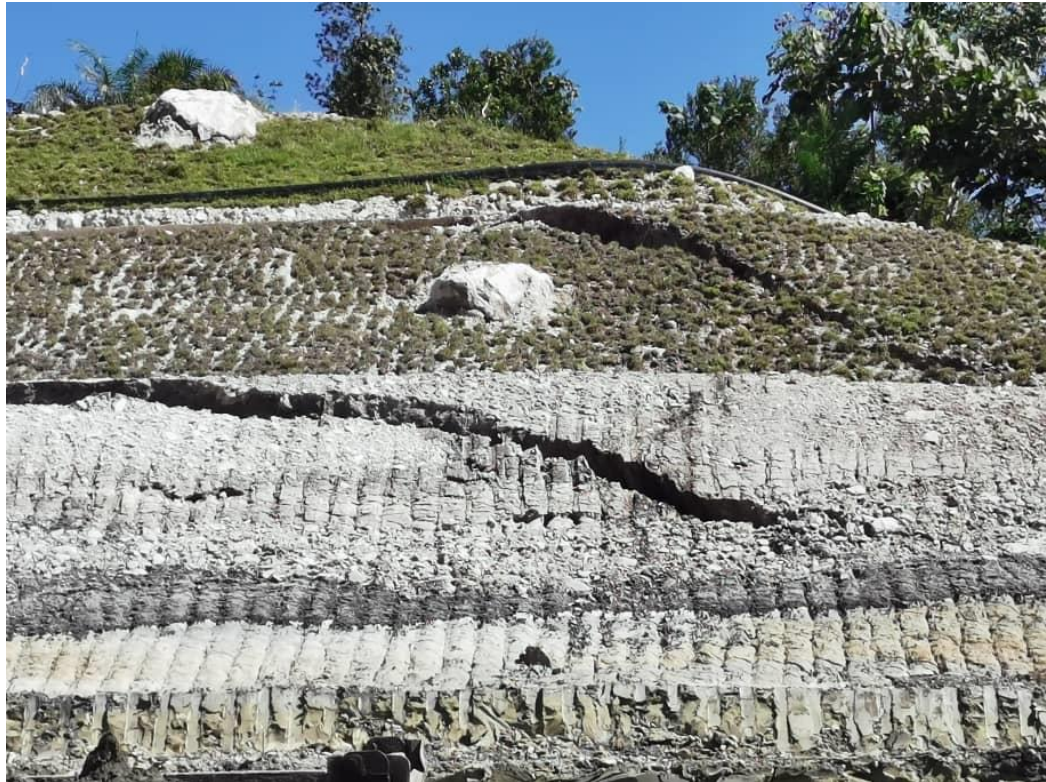
Figure 4.1: Movement Detected on Slope at Test Site 1. This Situation similarly Experienced at Test Site 2 And 3. ERT was Carried out on the Top Bench of the Slope
