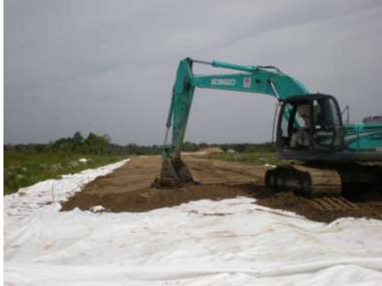
Figure 2.3: Installation of geotextile and sand platform (Photo taken at Sri Aman road construction site)
