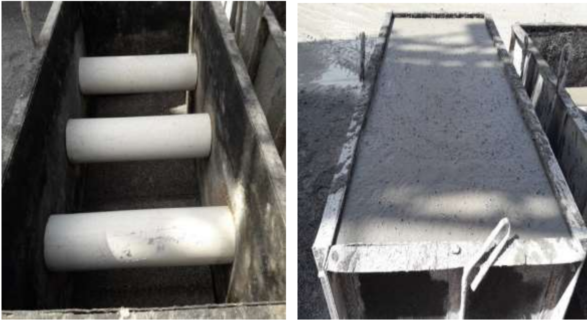
Figure 710: The casting of precast foamed concrete in mold
