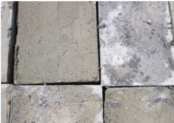
(d) Gap between shall less than 10 mm
