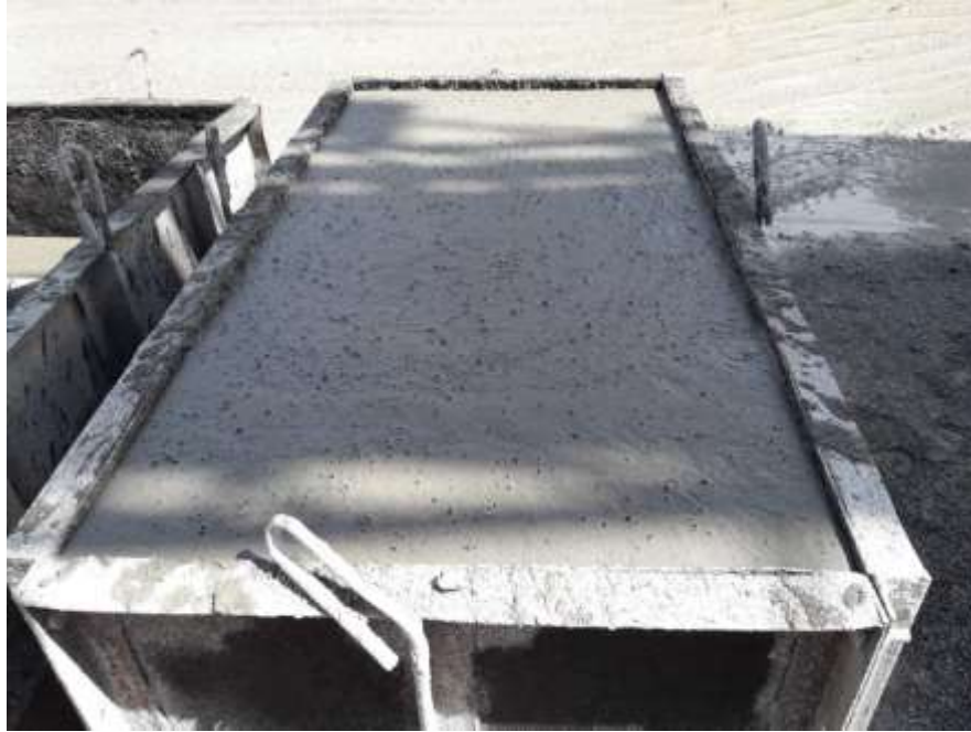
Figure 6.6: Foamed concrete produced by batching plant
