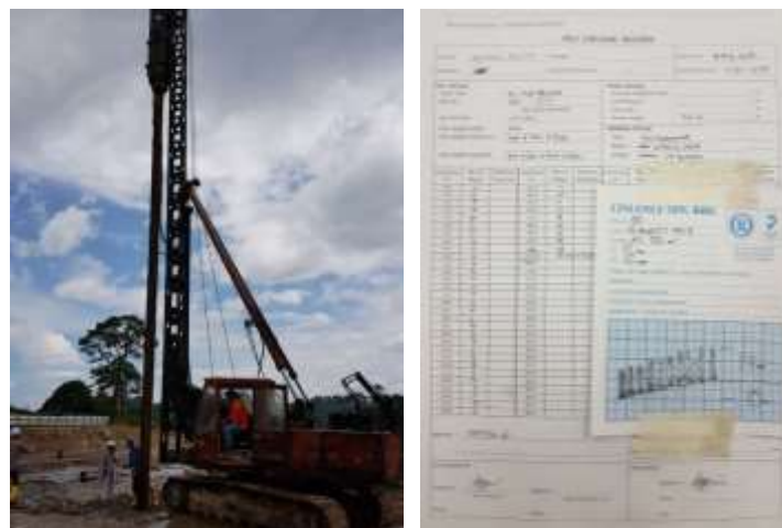
Figure 2.10: Installation of the pile at site and piling record (Photo taken at project site Santubong)
