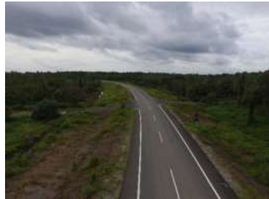
(f) Road completed
