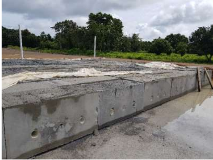
Figure 6.8: Foamed concrete foundation by new mixing technique
