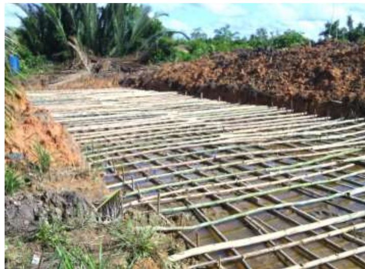
Figure 2.2: Bamboo mattress that has been tie together (Photo taken at Pusa road construction site)
