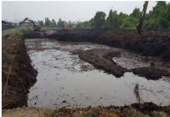
Figure 2.1: Unwanted peat soil has been excavated then filled with sand (Photo taken at Matang road construction site)
