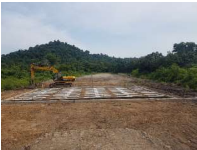
(a) UPVC Pipe installation
