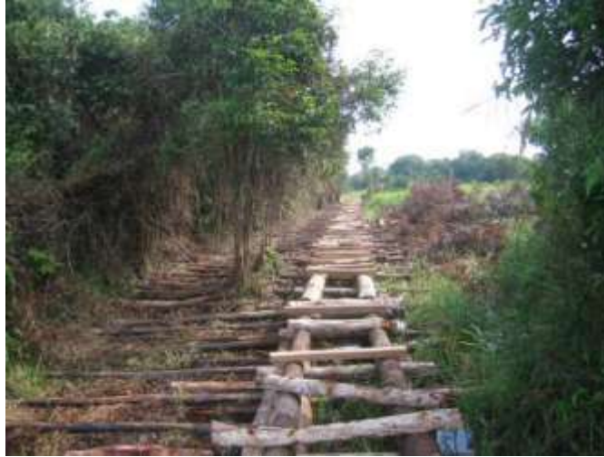
Figure 1.9: Floating timber track on peat area
