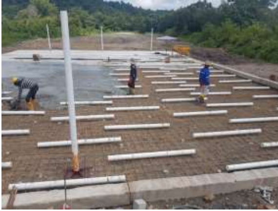
(c) Concreting the base
