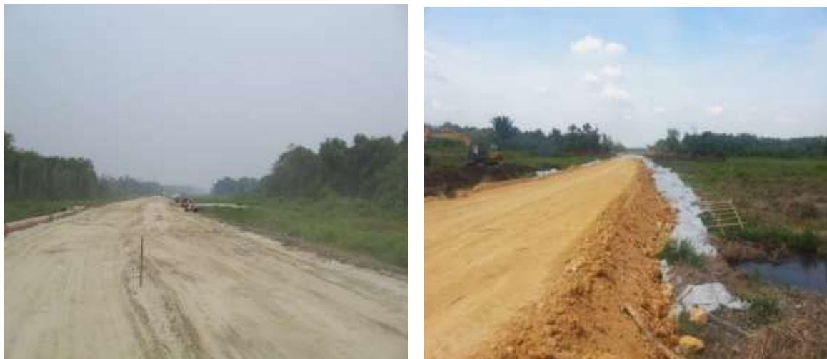
Figure 2.6: Sand filled to surcharge level (Photo taken at Samarahan road construction site)
