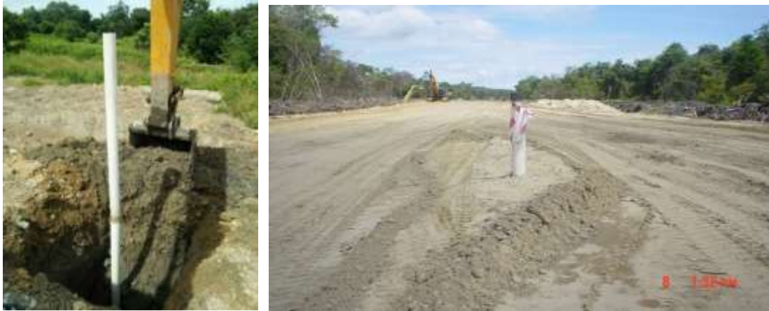
Figure 3.6: Monitoring of settlement after reaching the surcharge level by settlement plate (Photo taken at a road construction site at Samarahan)
