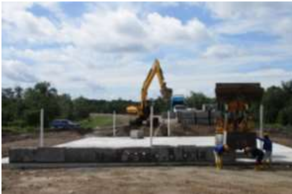
(e) Installation of Precast foamed concrete
