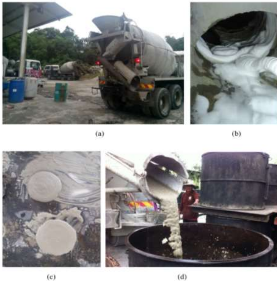
Figure 6.3: Big volume mixing in mixer truck; (a) mixer truck, (b) spraying the foam into the mixer truck drum, (c) slump measurement and (d) pouring into the formwork
