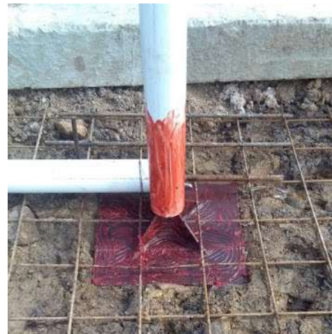
(b) Settlement Plate installation
