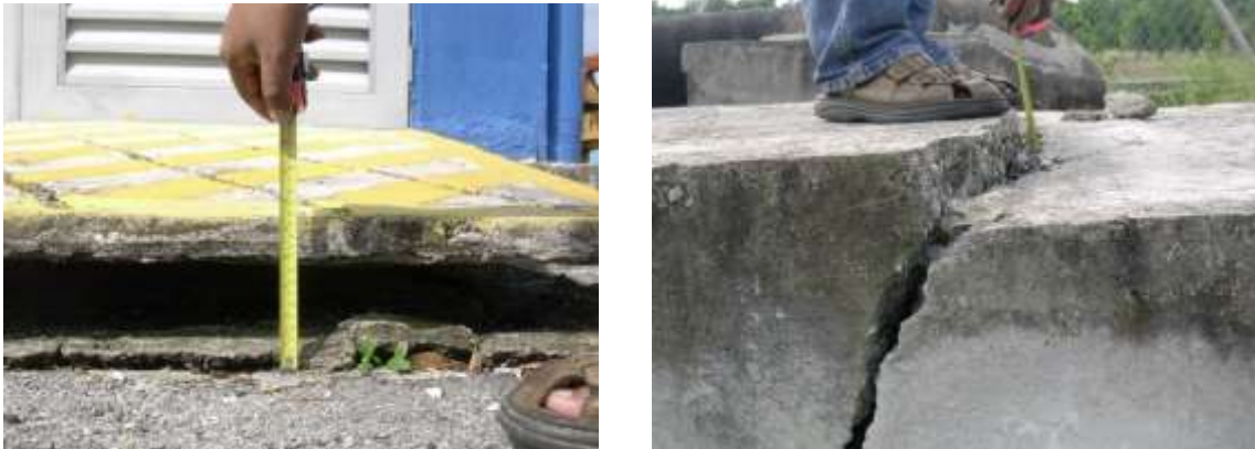
Figure 1.4: Settlement by water drain out
