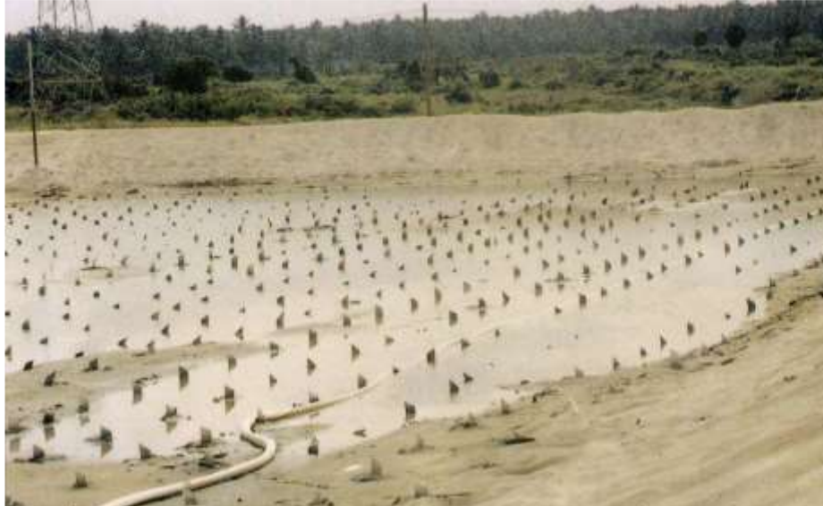
Figure 2.5: Installed PVD (Photo taken at Betong road construction site)
