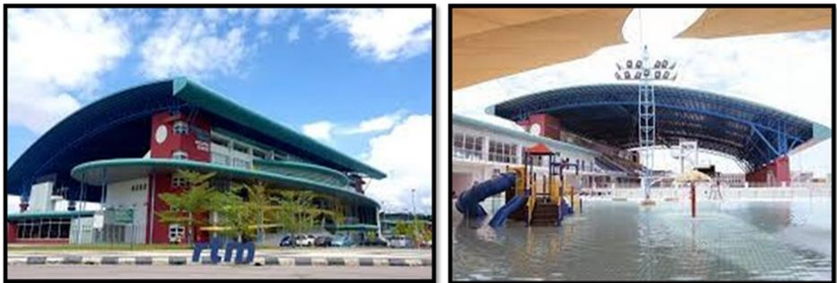
Figure 3.4: Pandelesa Rinong Aquatic Centre, Kuching
