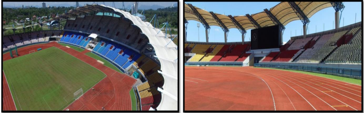
Figure 3.6: Sarawak Stadium, Kuching
