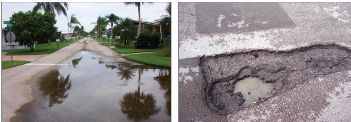
Figure 1.2: Poned Water and the Formation of Pothole
