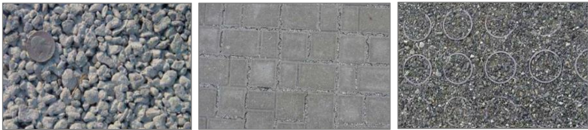
(a) Pervious Concrete
