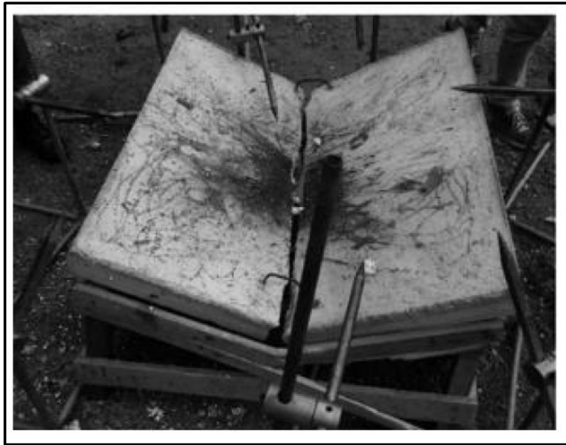
Figure 1.3: Slab failure under blast loading (Mendonça et al., 2018).
