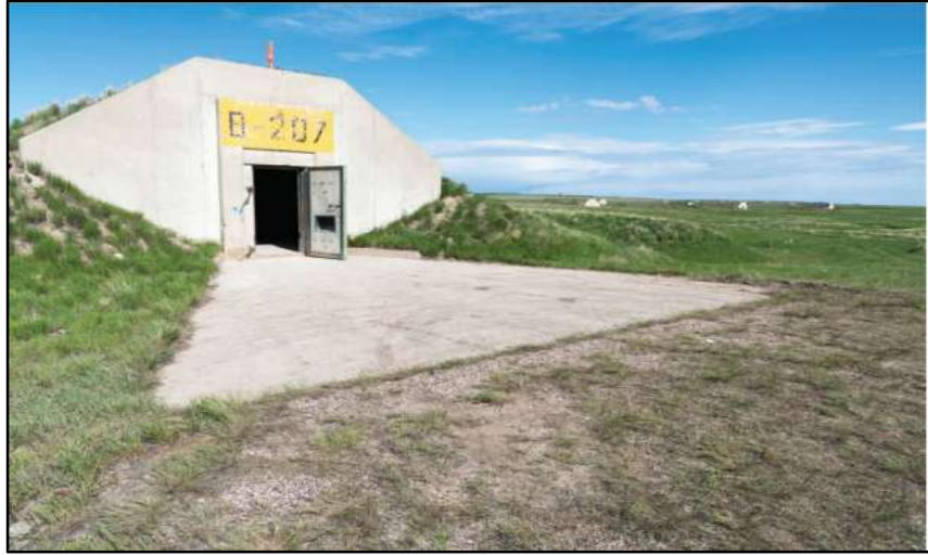
Figure 2.5: A bunker in South Dakota (Garrett and Klinke, 2019).
