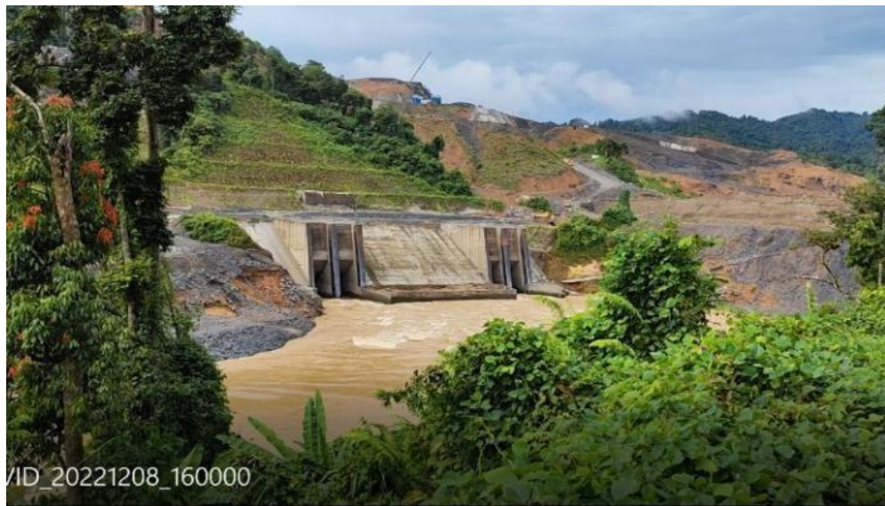
Figure 4.2: The tunnel system for the Baleh HEP Dam
