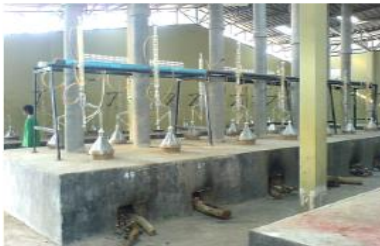
Figure 2.6: Conventional distillation plant with wood fire stoves (Pakamas, 2012)
