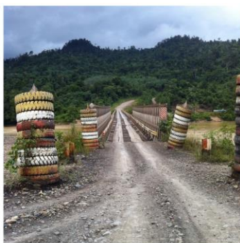
Road construction to midstream area (02/09/2015, 0915)
