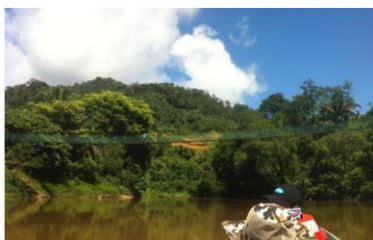
A bridge connecting Long Moh to their school (29/07/2015, 1159)
