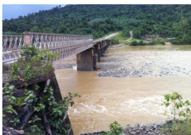
Long San's Bridge connecting downstream area to midstream area (12/01/2016, 0906)
