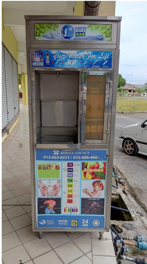
WVM without dispensing area cover and situated near an open drain
