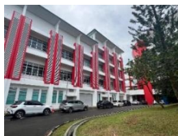
(c) Street view of the Mechanical Department block
