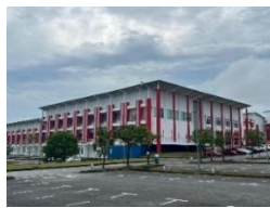
(a) Street view of civil engineering lab
