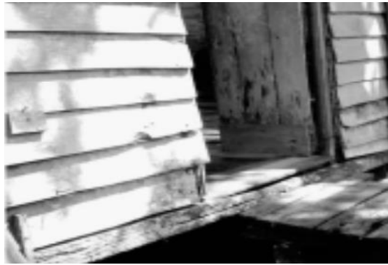
Figure 2.5 The susun sirih wall arrangement (Zain, 2012).
