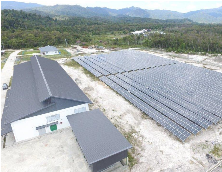
Figure 2.2: Centralized Solar Hybrid System in Bario, Sarawak (Borneo Post, 2016).
