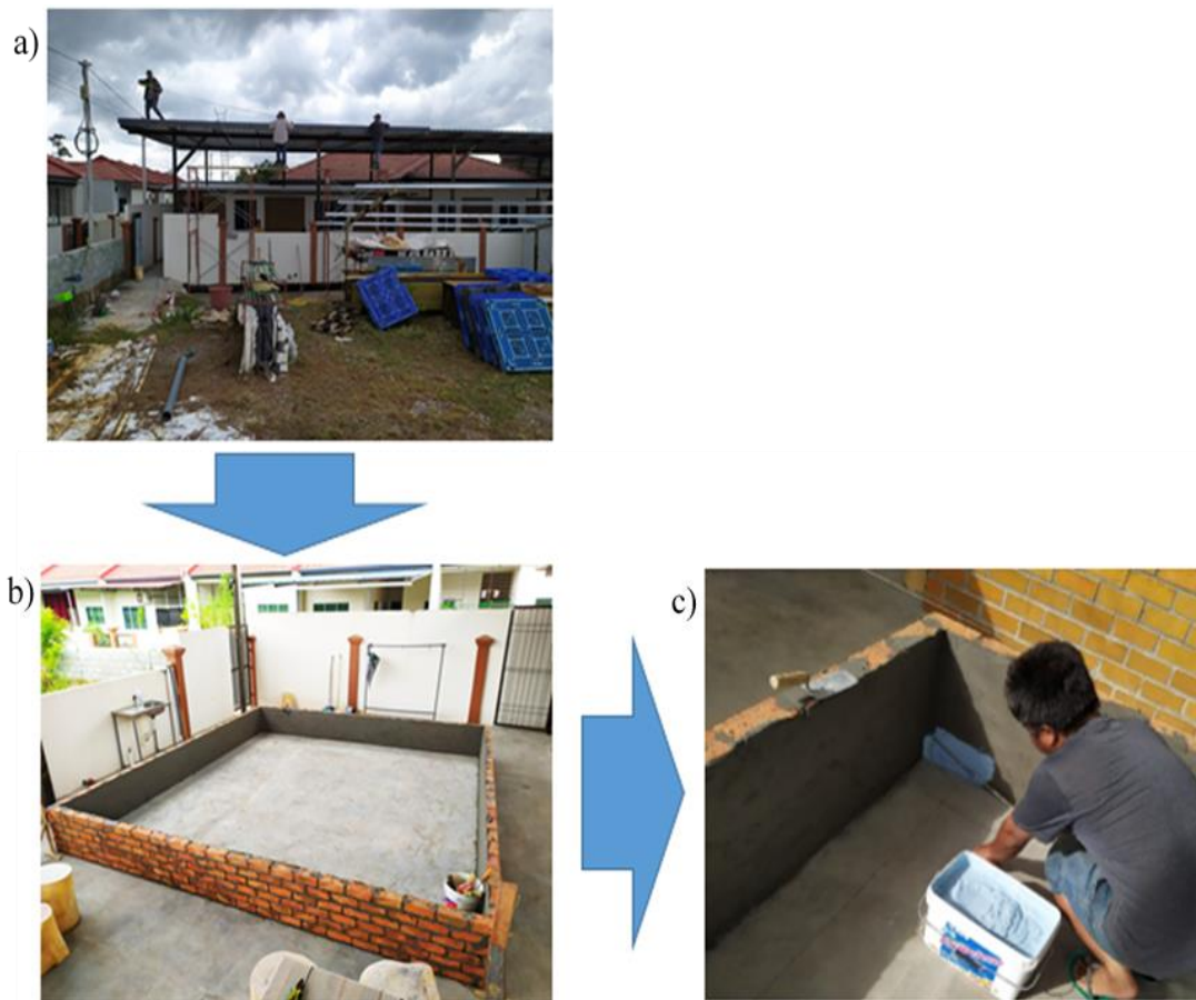
Figure 3.6: Construction of Home-Based StormPav OSD, a) Delineation of Roof, Installation of Roof Gutter and Downpipe, b) Brick Layering and c) Water-proof Treatment
