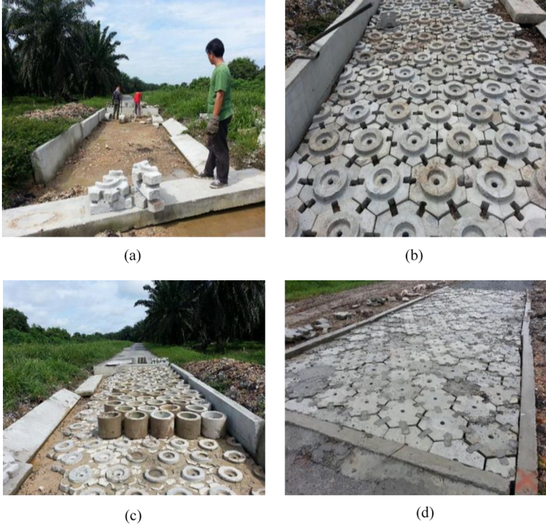
Figure 2.9: Assembling of StormPav Road, (a) Levelling of Soil Level, (b) Arranging of Bottom Plates, (c) Arranging of Cylinders, (d) Arranging of Top Plates (Mah et al., 2018c)
