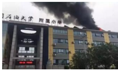
(d) Rooftop Photovoltaic Power Station of a Primary School
