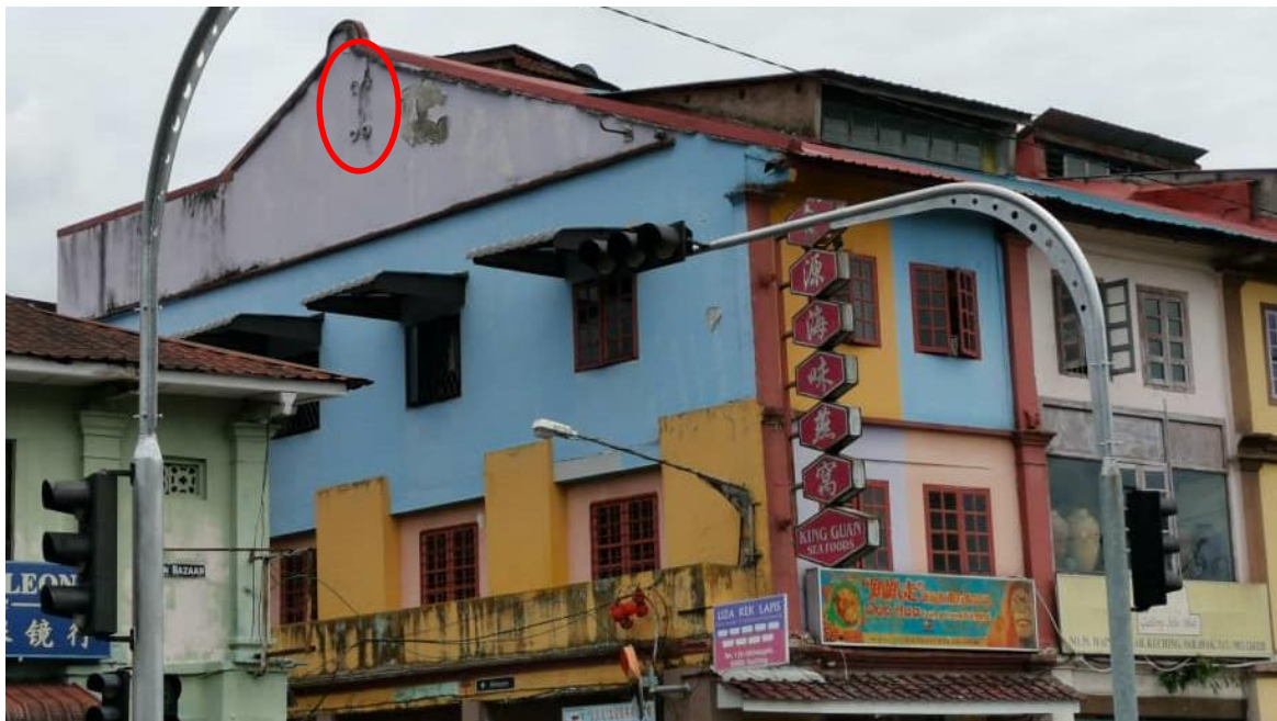
Figure 2.2: One of the URM Buildings at Kuching Waterfront With Wall Anchorages
