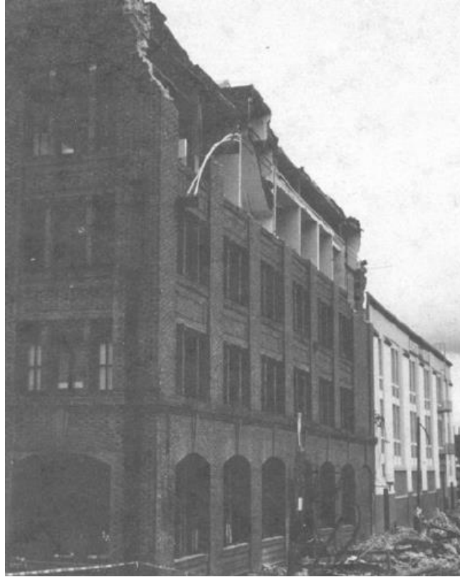
Figure 1.3: Out-Of-Plane Failure of URM Top-Storey Wall at San Francisco, Loma Prieta Earthquake (Bruneau, 1994)
