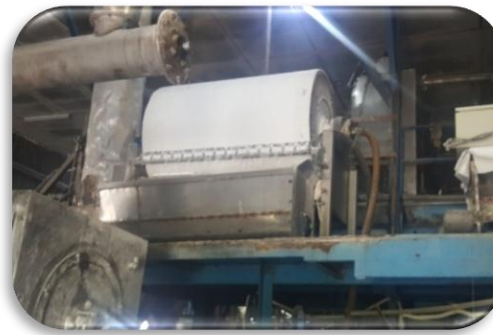
Dewatering and drying
