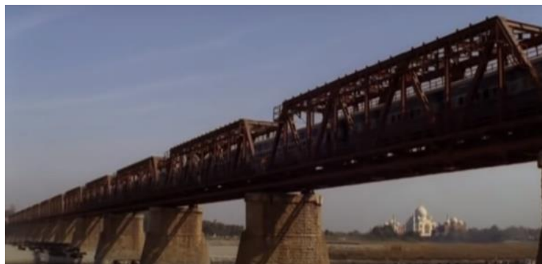
Figure 4.20: Railway Bridge as a Symbol of Colonial Infrastructure
