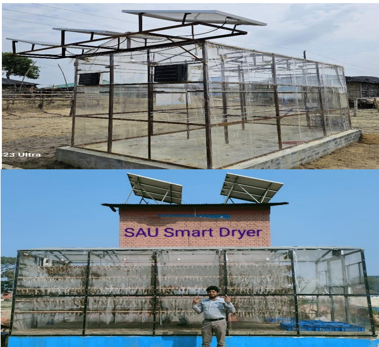
Figure 4.3: Installation of hybrid solar dryer
