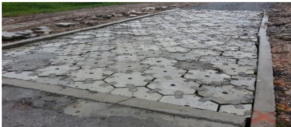
Figure 2.18: Pilot study of StormPav Green Pavement in Kampung Mang (Mah et al., 2018c)
