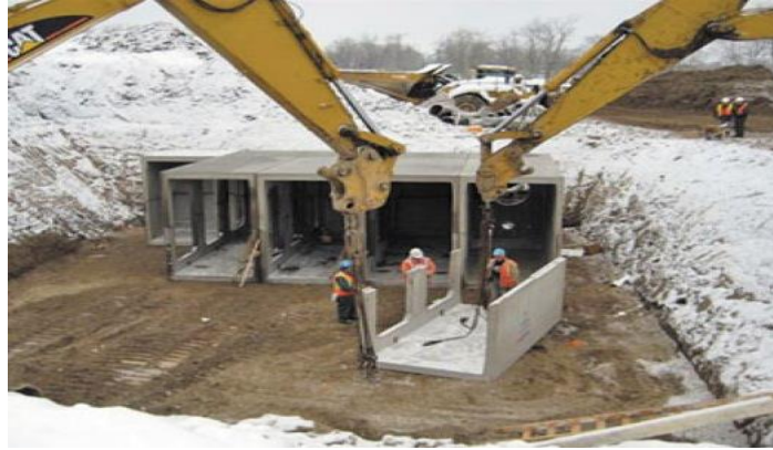
Figure 2.14: Installation of Precast StormTraps (Kenter, 2011)
