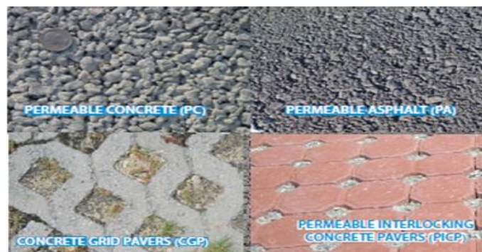
Figure 2.4: Types of Permeable Pavements (Hunt & Collins, 2007)
