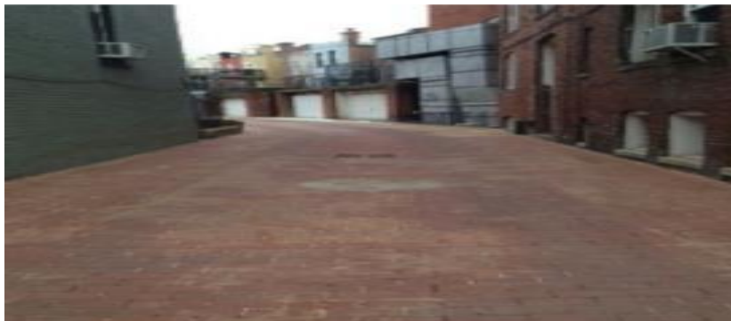
Figure 2.8: Permeable Road of the Bloomingdale Project (District Department of Transportation, 2014)
