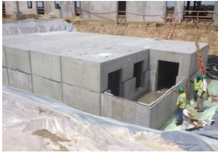
Figure 2.13: Installation of StormCapture Beneath the Carpark (Old Castle Infrastructure, 2018)
