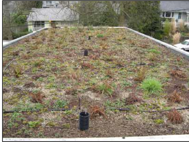
Figure 2.3: An extensive green roof at the Ross Park Shelterhouse in Seattle, United State (Seattle Public Utilities, 2012)
