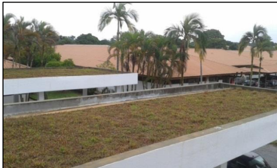
(a) Condition of green roof
