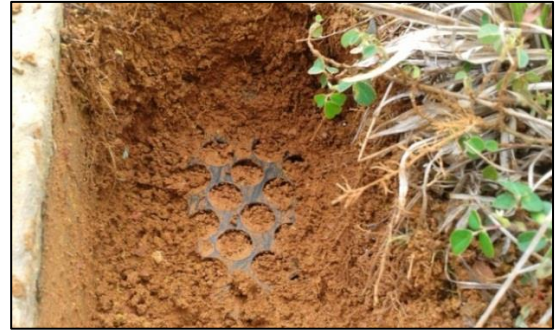
(b) Geosynthetic sheet drain
