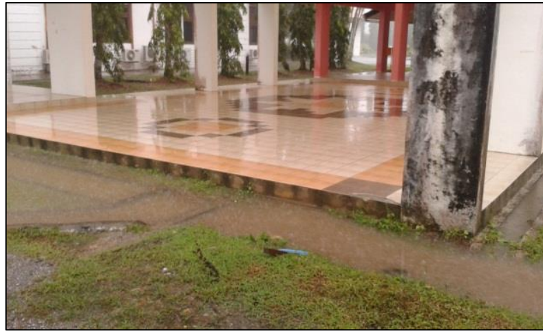
Figure 3.8: Overflow of stormwater from swale into outlet of downspout pipe is observed during a heavy event on 21 December 2014.
