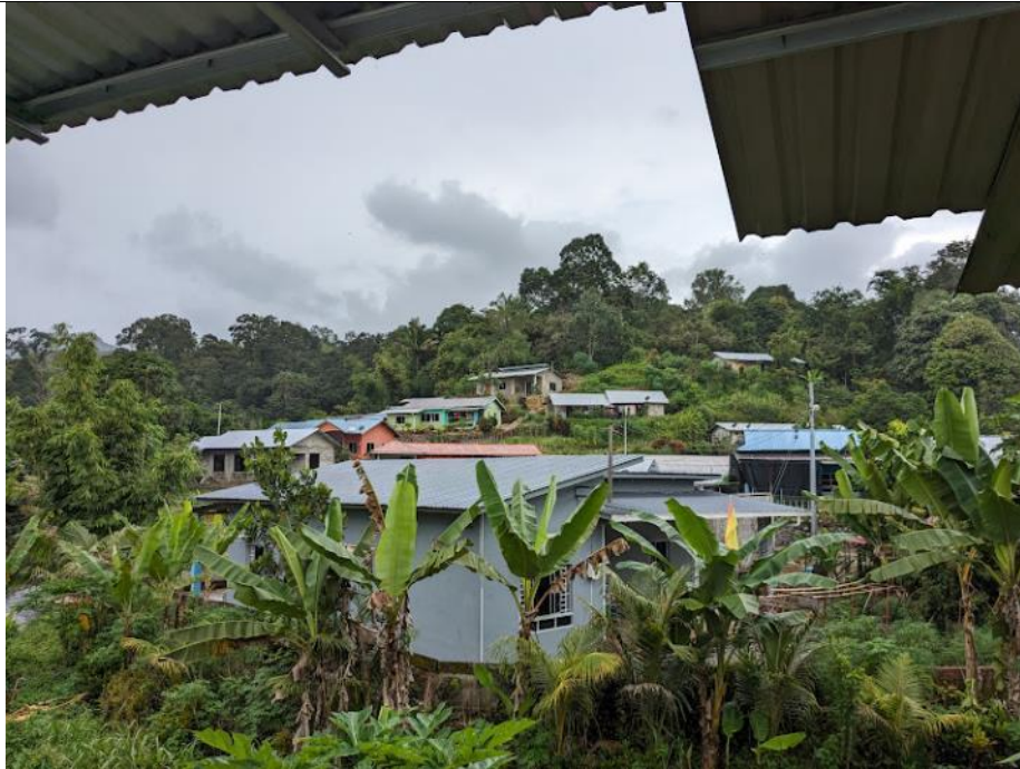
Figure 27: Kampung Tangga Mawang Group 4 Site Conditions
