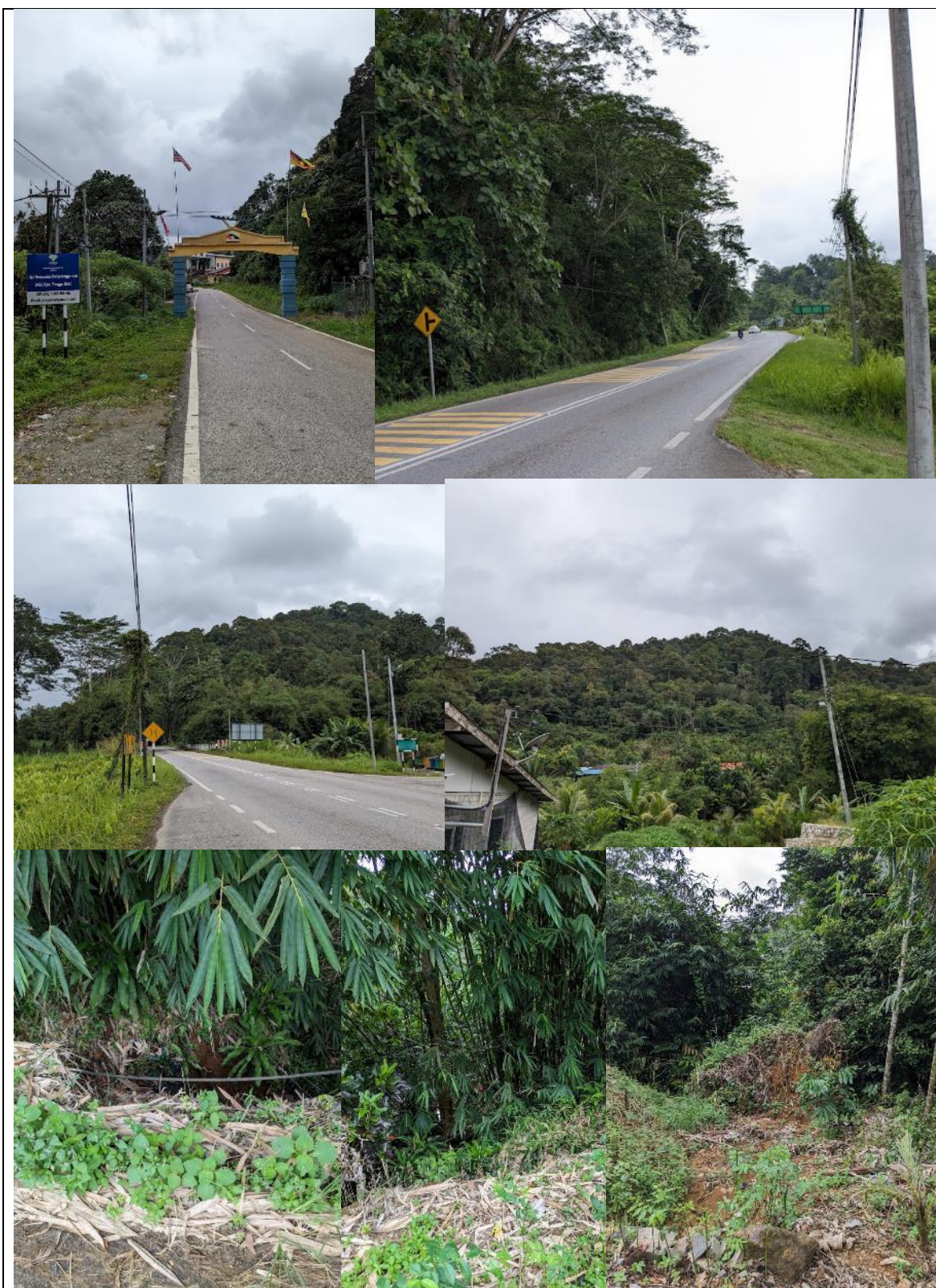
Figure 27: Kampung Tangga Mawang Group 1-3 Site Conditions
