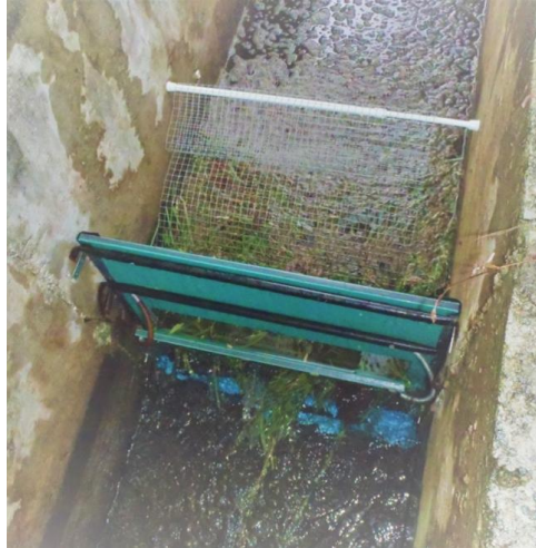
Figure 4.18: The leaf-gate was stuck due to large amount of leaves passing through the trash trap
