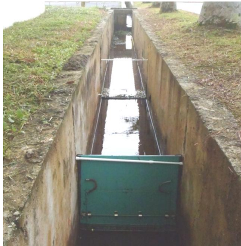
Figure 4.19: The trash trap was installed 2.5m away behind the gate
