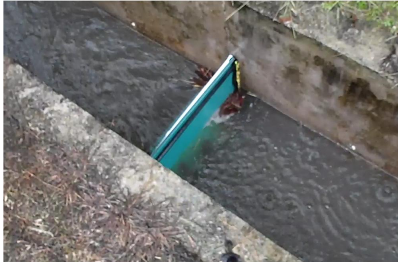
Figure 4.22: Leaves get stucked at the gate frame
