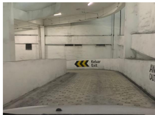
Going down through a dangerous slope 2
