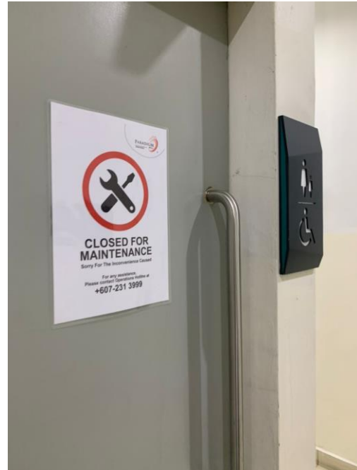
Malfunction toilet for disabled people and children
