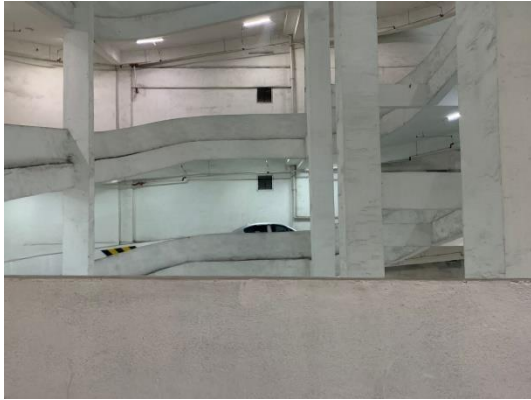
Going down through a dangerous slope 3
